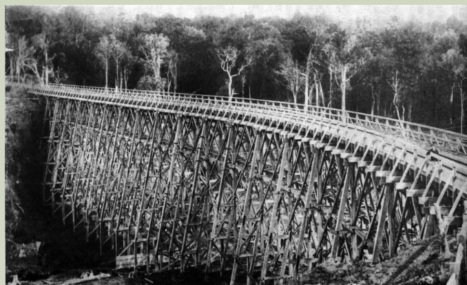
Above: The settlers first built the Mangarangiora viaduct, near Ormondville, entirely of wood. Below: The steel viaduct in 2011.
